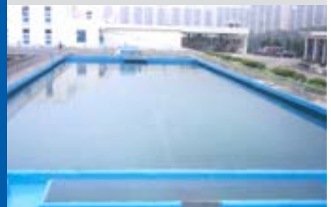
Cem-Kote Flex ST - water treatment facility, Daejeon, Republic of Korea
