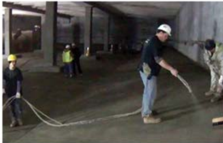
Cem-Kote Flex ST spray and brush application, Streetsville, Ontario, Canada
