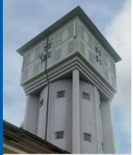
Cem-Kote restoration and waterproofing of water tower, Josefov, Czech Republic
