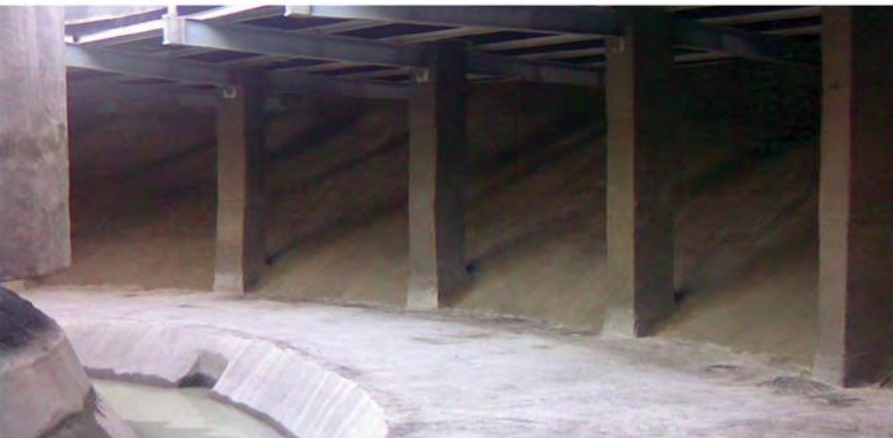
Cem-Kote Flex ST used to restore and waterproof WTP in Calarasi, Romania
