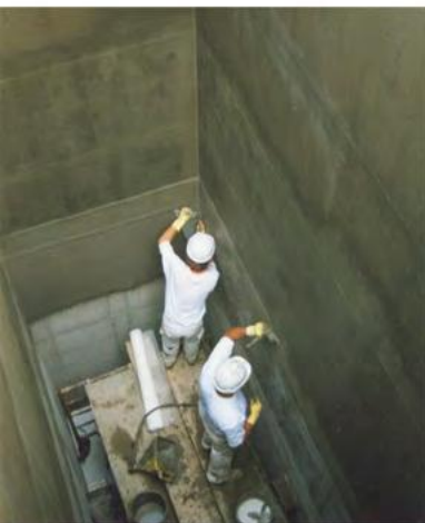
Installation of Cem-Kote Flex ST with Reinforced Fabric HD throughout (entire surface), Kingsford, Ontario, Canada
