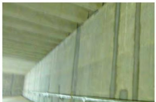
Cem-Kote Flex ST with Reinforcing Fabric HD to provide long term crack bridging, Mississauga, Ontario, Canada
