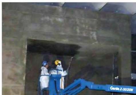
Cem-Kote Flex ST applied to walls and slab, Herridge WTP, Mississauga, Ontario, Canada
