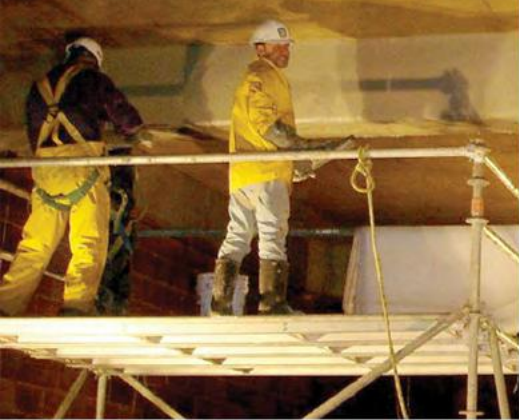
Cem-Kote Flex ST and Reinforcing Fabric HD applied over a high number of cracks in the beam, Guelph, Ontario, Canada
