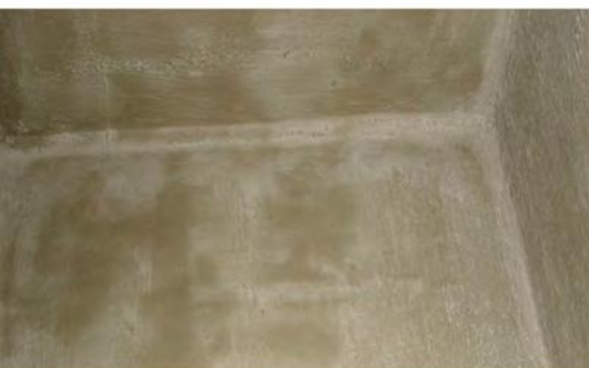
Horizontal and vertical coves using Fibre-Patch OV, Cem-Kote Flex ST and Reinforcing Fabric HD, Brantford, Ontario, Canada
