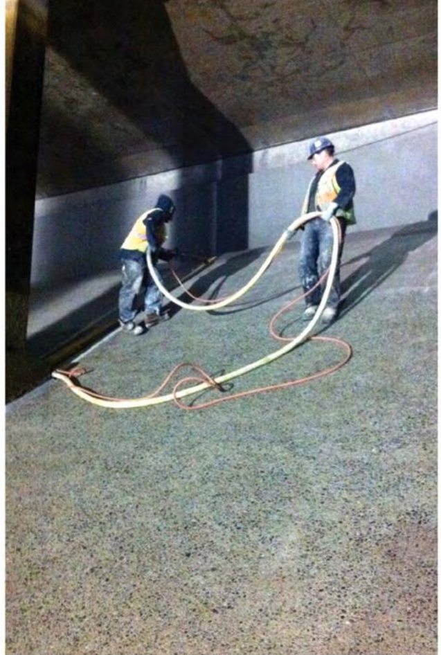
Spraying Cem-Kote Flex ST , Whaley WTP, Vancouver, British Columbia, Canada
