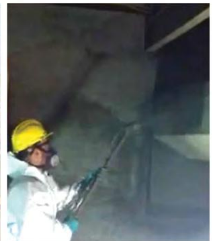
Spraying of Gem-Plast TC to repair and level deteriorated concrete surface, Niagara, Ontario, Canada
