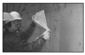
Apply second, stiffer consistency, coat of *Cem-Kote CW Plus* into the wet slurry by trowel. Keep wet edge. Do not build up a layer thicker than 6 mm (1/4 in). In new construction, *Cem-Kote CW Plus* is dry-sprinkle applied onto the surface of the freshly poured slabs (after the concrete starts to reach initial set) and is power trowel finished.
