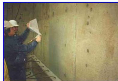
**Figure 38:** Spray application of Cem-Kote Flex ST. This simple hopper gun equipment for later changed for a more efficient pump.
