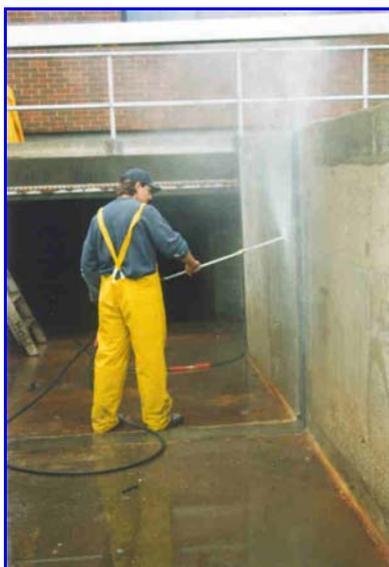
**Figure 11:** Surface preparation using 3,500 psi (23 MPa) water
