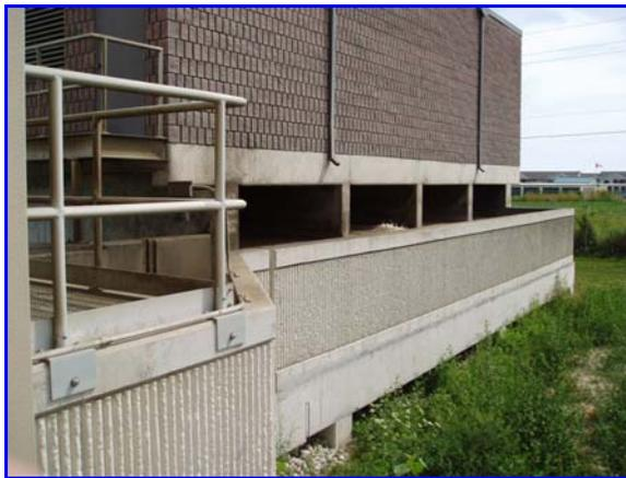
**Figure 34:** Exterior view of the grit channels after 3year use. No leaking is visible.
