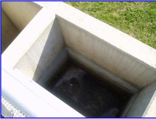
**Figure 27:** View into the grit channel wells, waterproofed with Cem-Kote Flex ST and reinforced with the Reinforcing Fabric HD. Cem-Kote Flex ST is the light grey material in the well.
