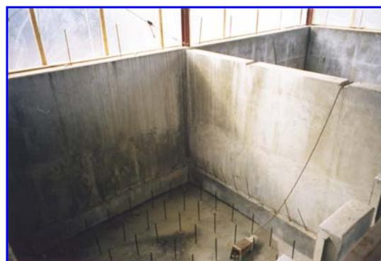
**Figure 40:** Cem-Kote Flex ST waterproofed tank
