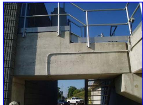
Figure 15: North side view of the grit channel (trough) – no leaks are visible.
