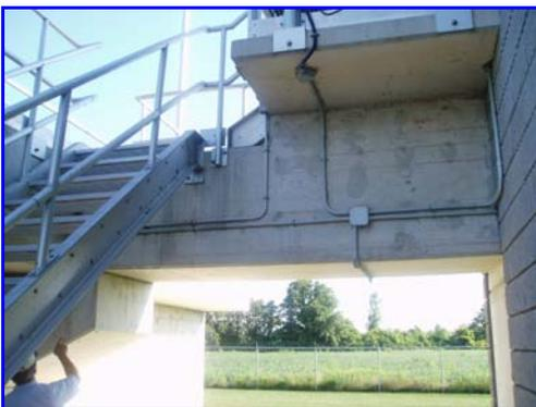
Figure 14: South side view of the grit channel (trough) – no leaks are visible
