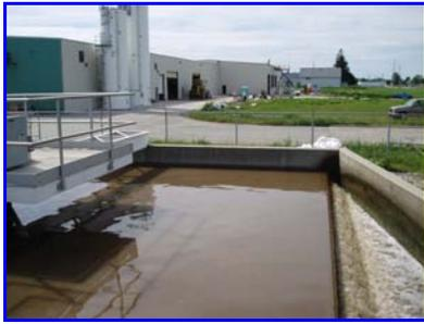
**Figure 31:** The same area as shown in Figure 29, during inspection in August 2005. No deterioration, delamination or cracking of Cem-Kote Flex ST observed.
