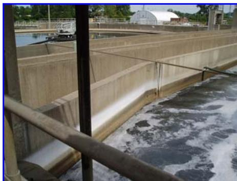
**Figure 10:** The channel, the same as shown in Figure 9 after 12 years. There is no deterioration, cracking or de-bonding of Cem-Kote Flex ST. Deposits of salts in the area where the alum is discharged form the white discoloration.
