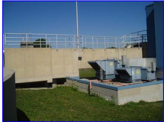
**Figure 28:** The "north side" view of the grit channel trough) at the pump station – no leaks are visible
