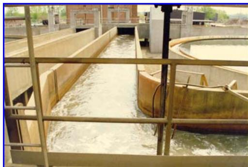
**Figure 9:** The continuously used channel before the repair – note the rail s where the alum is introduced into the stream – concrete deterioration at this area was approximately ¼ to 3/8 in (6 – 9 mm) deep
