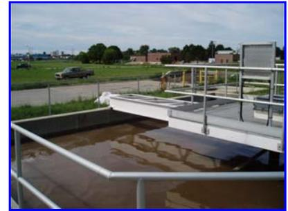
**Figure 33:** The same tank as shown in Figures 29, 31 32 – a different view – again no deterioration, delamination or cracking of Cem-Kote Flex ST observed,
