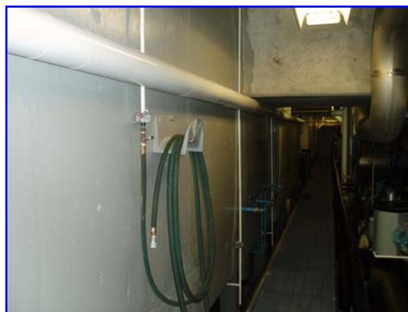
**Figure 42:** Exterior wall of the tanks – no leaks are visible
