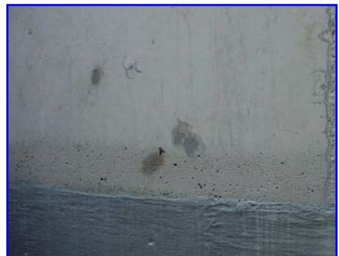
**Figure 30:** Cem-Kote Flex ST, brush applied – please note the prepared surface after a high-pressure wash, just above the Cem-Kote Flex ST.
