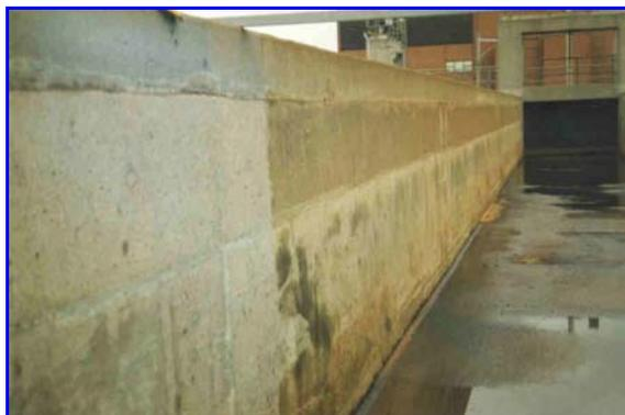
**Figure 12:** The channel surface after surface preparation, prior to application of Cem-Kote Flex ST
