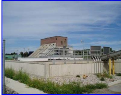
**Figure 32:** The same tanks as shown in Figures 29, 31 and 33 – outside view. There are no leaks visible in the walls of the tank.
