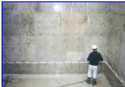
**Figure 37:** Cleaning the surface of the tanks prior to application of Cem-Kote Flex ST
