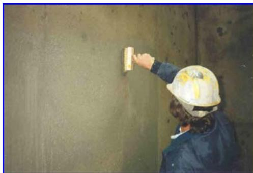
**Figure 39:** Brushing of Cem-Kote Flex ST to eliminate pinholes.
