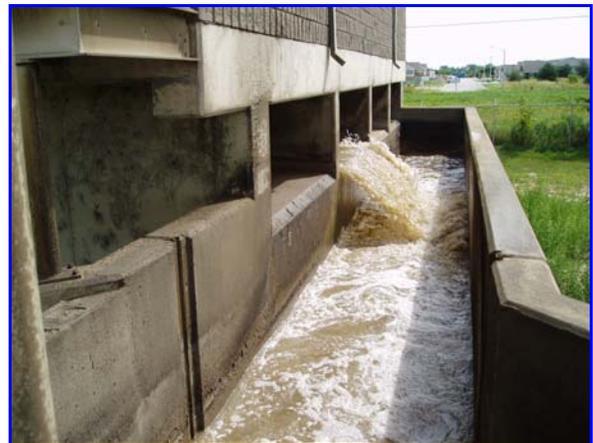
**Figure 35:** Interior view of the grit channels after 3 years of use. No deterioration due to chemical attack or abrasion, delamination or cracking was observed
