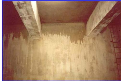
**Figure 44:** The wall and ceiling was also treated with two coats of Cem-Kote Flex ST.
