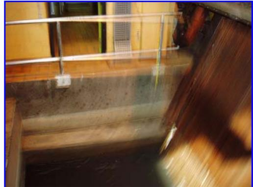
**Figure 6:** Chambers at the primary filtration station – 12 years later – no visible deterioration, cracking or de-bonding of Cem-Kote Flex ST was observed, just some discoloration
