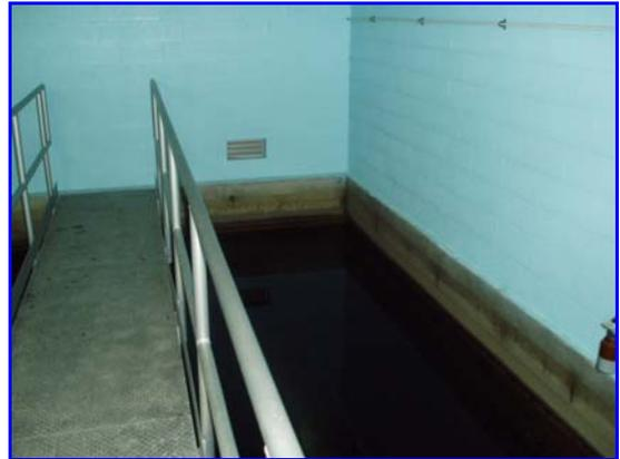
**Figure 46:** Fibre-reinforced Gem-Crete CR,  $\frac{1}{2}$  in (12 mm) thick, applied to the walls and bottom of several concrete tanks.
