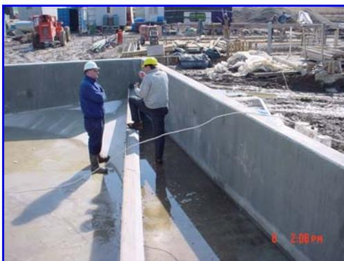
**Figure 29:** Inspection of Cem-Kote Flex ST application in 2002
