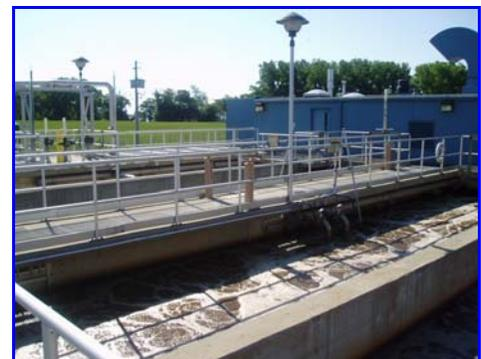
**Figure 20 (right):** Aeration tanks – the “blue” building contains the mechanical rooms
