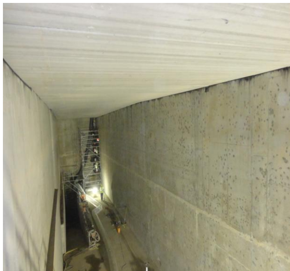
Figure 2. Tank 1A of the facility
