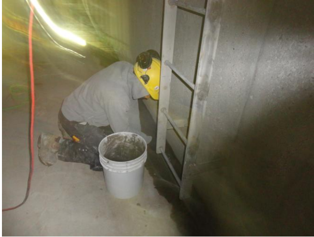
Figure 4. Installation of the corner “coves”
