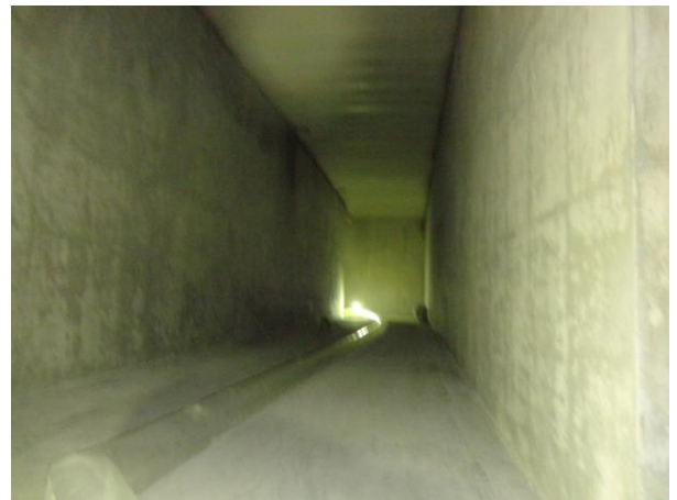
Figure #7. Finished application of Cem-Kote Flex ST in Tank 1A
