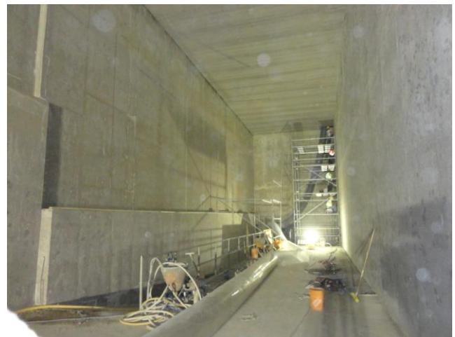
Figure 3. Tank 1A of the facility
