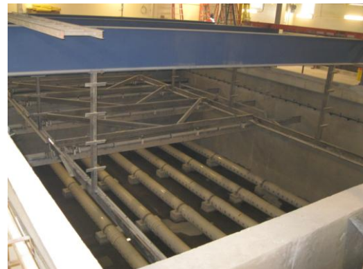
Figure #2: Tanks - Cem-Kote Flex ST applied
