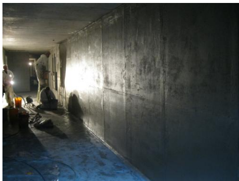
Figure #3: Application of Cem-Kote Flex ST and the Reinforcing Fabric HD
