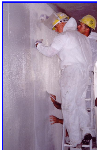
Placement of the Reinforcing Mesh HD and spray application of Cem-Kote Flex Plus
