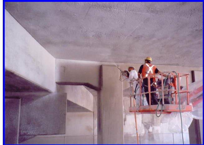
Spray application of Cem-Kote Flex Plus
