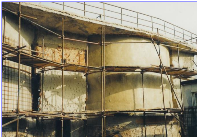
Wet shotcrete process was used to structurally repair the tanks
