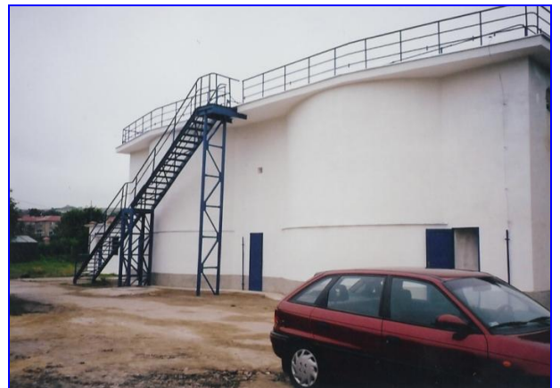
Finished restoration – the interiors of digester tanks were coated with Cem-Kote Flex CR and the exterior structure was coated with Cem-Kote ST White
