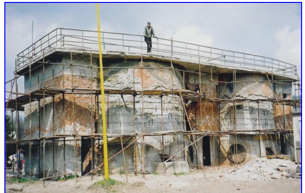
Structure with digester tanks before restoration
