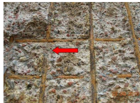
Figure 2 - right: the “top” reinforcing steel in some places was completely corroded
