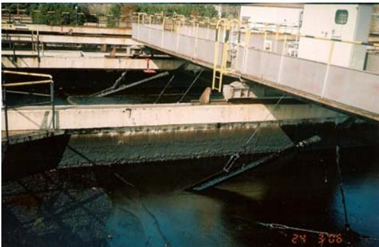
**Figure 5.** Oil and grease deposits on the surface of concrete tanks
