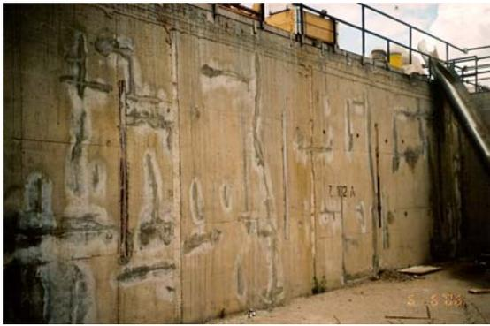
**Figure 11.** Cracks filled with fibre reinforced mortar bonded with polymer modified cement slurry to the polyurethane seal
