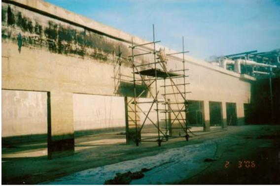
**Figure 7.** Sandblasting after chemical cleaning
