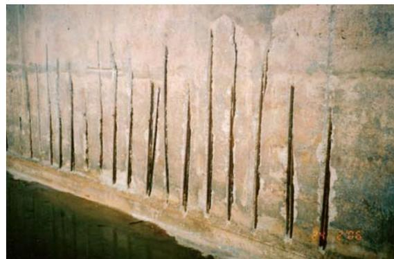
**Figure 4.** Delaminating concrete due to corrosion of reinforcing steel
