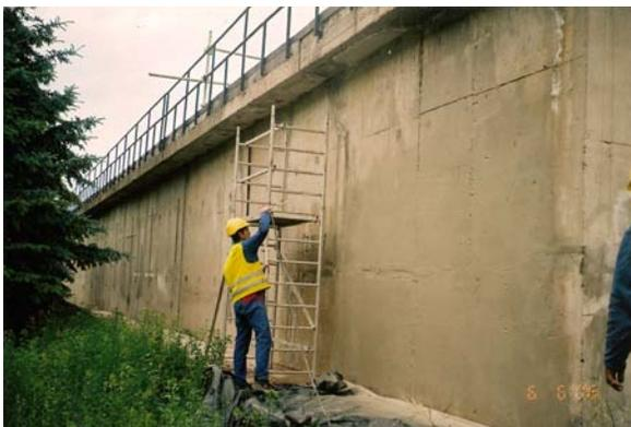
**Figure 17.** Application of one component polymer modified cement coating to the exterior of the tank
