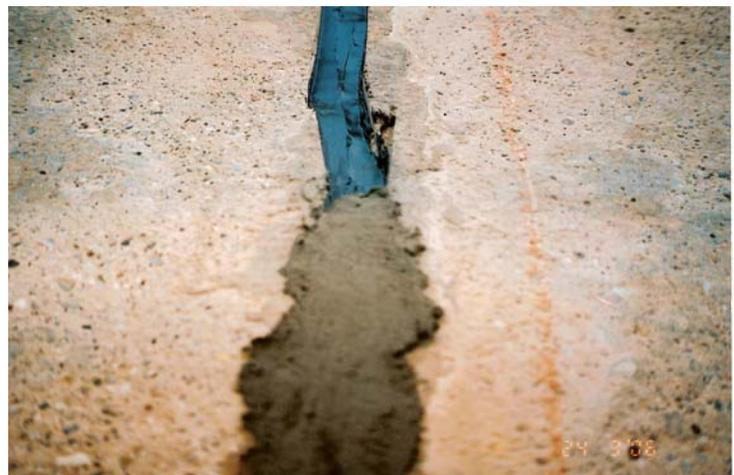
**Figure 10.** Cracks filled with fibre reinforced mortar bonded with bonding agent to the polyurethane seal
