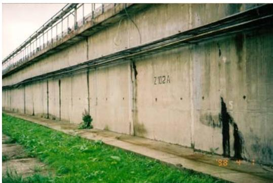
**Figure 3.** Leaks in concrete tanks
