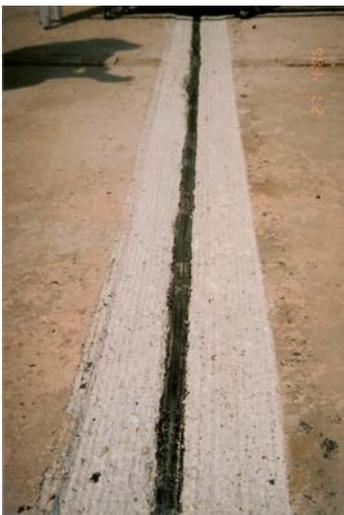
**Figure 13:** Expansion joint after milling, before placement of the sealant and the rubber sheet.
